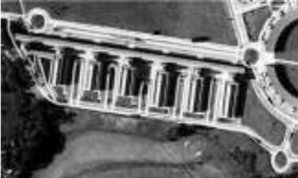
Fig. 12 Aerial picture of the circuit used in the tests. In the left of the image, a portion of the road is shown between the building and an area covered with trees, where GPS measurements are difficult
